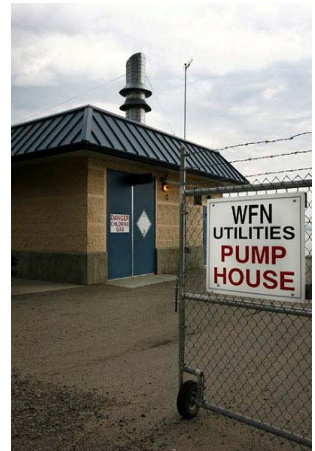
IR #1—Pump House
