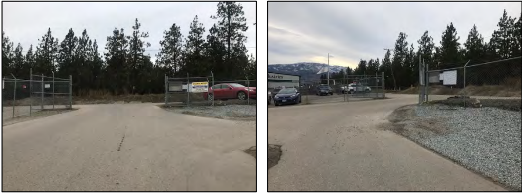
Gate 1 – Russell Building Entrance: 3500 Red Cloud Way (Existing Gate)
