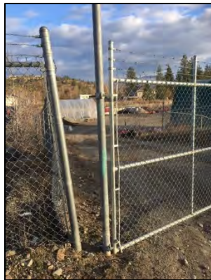
Vehicle Gate 2 – Yard Entrance: 3255 Red Cloud Way (Existing Post)
